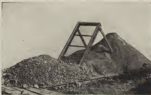
FIG. 11.—A slanting screen can be made to separate the sand from the coarse material in bank-run gravel, making possible a great improvement in the quality of the concrete produced.
